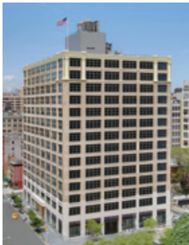
Top: 255 Greenwich Street Bottom: 250 Hudson Street
